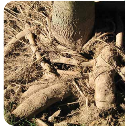
Performing a Root Collar Excavation using an Air Spade can reveal girdling roots. If they are left uncorrected, these circling roots can damage the stability of a tree's root system and restrict the flow of nutrients to the trunk.
